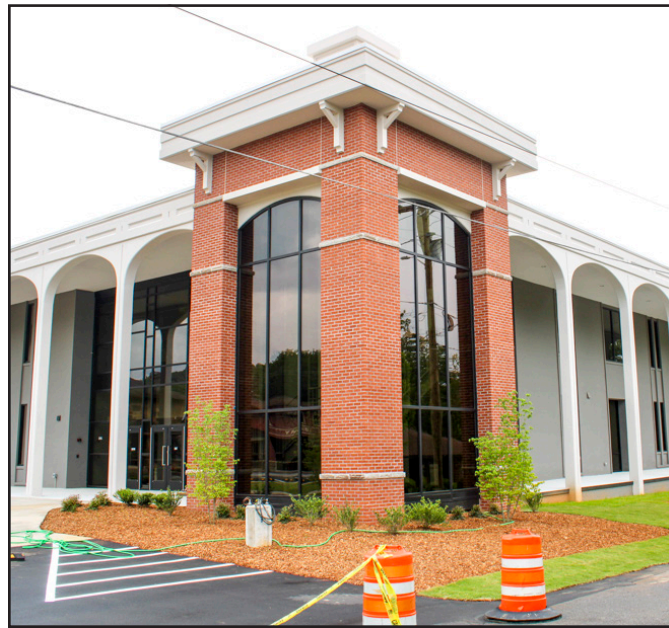
The newly renovated Towns County Courthouse will fully open in the middle of June, to feature two public Open Houses next week. Photo by Lowell Nicholson
